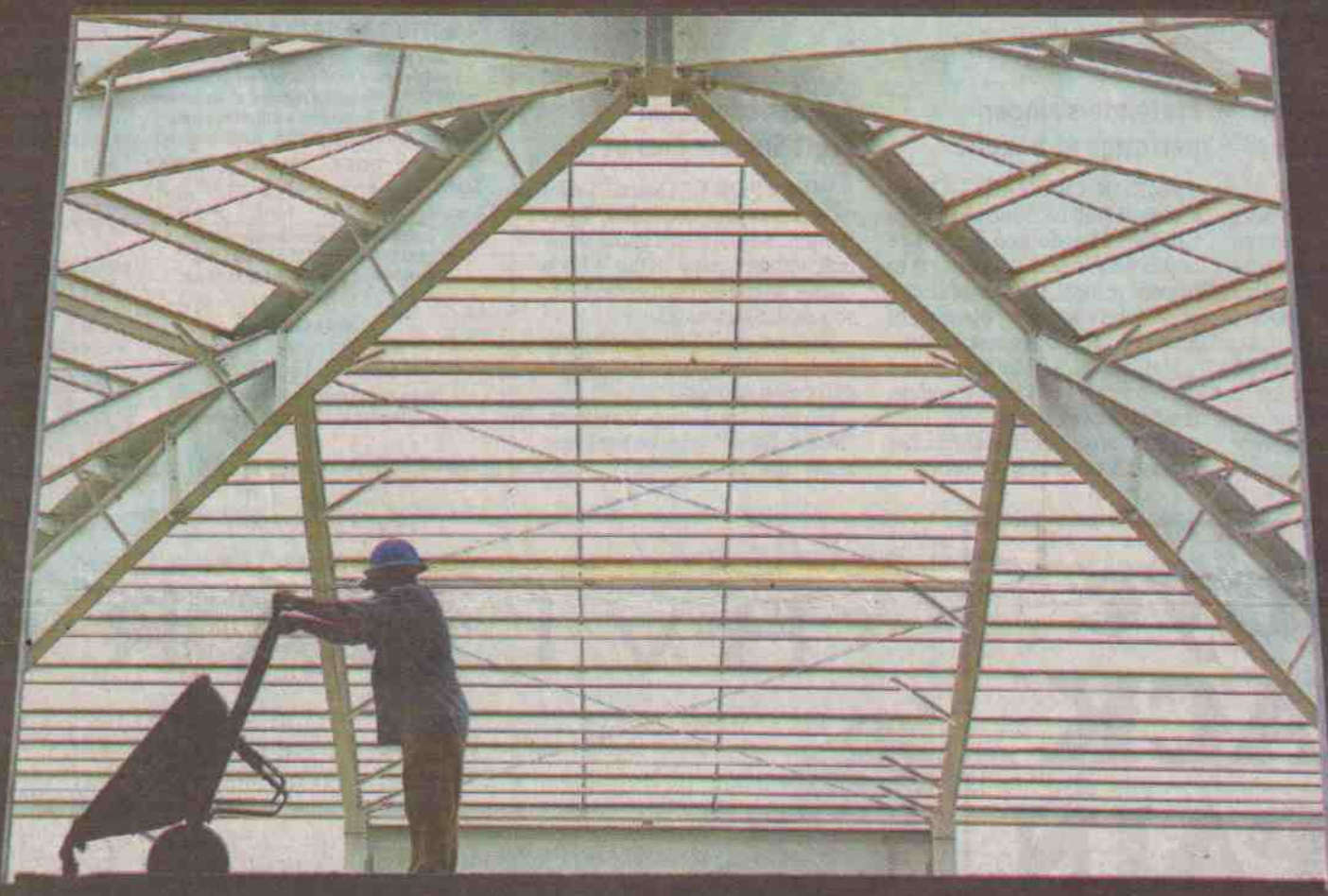
Tradesman Joe Soliz spreads mortar on the second floor of the food arena at the Naples Big Cypress Market Place on Sept. 7. The 87,000-square-foot shopping and entertainment center on U.S. 41 East in East Naples is scheduled to open in November. David Albers/Staff (2)
